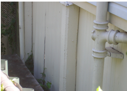
Illustration 5: Photo showing rotten and deformed timber of asbestos ridden derelict hovel.
