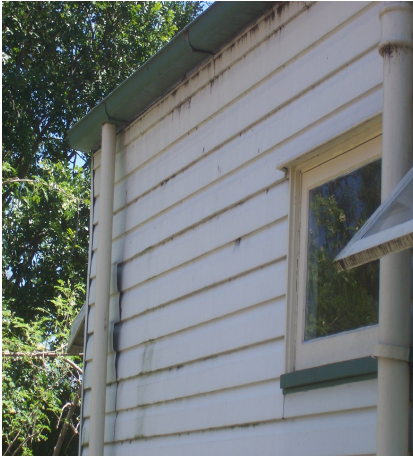
Illustration 4: Photo showing loose cladding as there is nothing substantial beneath to which cladding can be secured.
